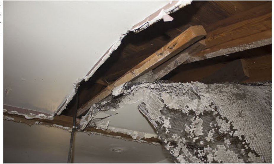
The roof was also modified across time and in this picture the metal lath can be seen, this modification probably took place under the major renovation held in the Howe Mansion in 1958.
