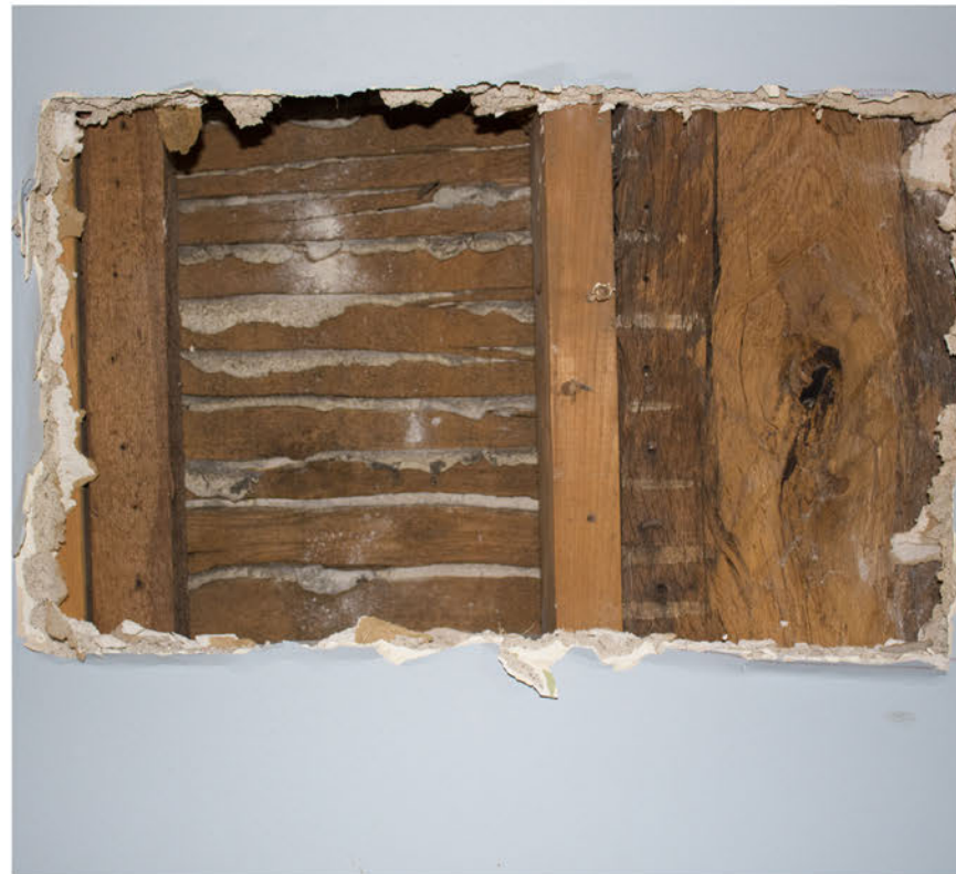
Detail. Original lath in the wall dividing the main volume and the South wing.
