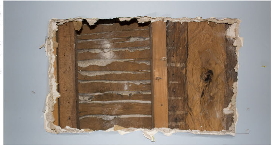
Photo where the original wood lath can be seen, the opening was done in the same room where the fireplace was added in the main two levels volumes but in the common wall with the right volume. The original wood lath is from the side of the right side volume and a “modern” gypsum board is in the side where the picture was taken from. This modification also probably took place in the major renovation undertaken in Howe Mansion in 1958.
