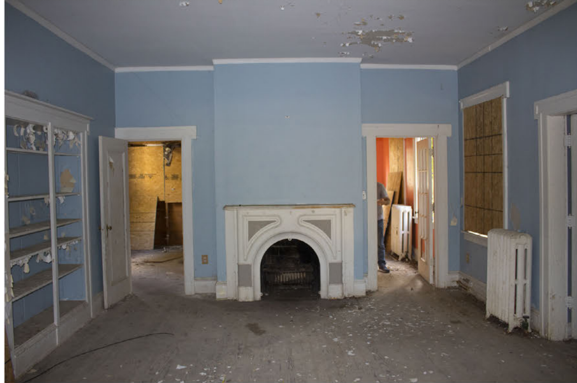
Photo of the current condition in the groundfloor of the main volume where a victorian fireplace was added, probably at the end of XIX Century with the construction of the New Mansion across the street.
