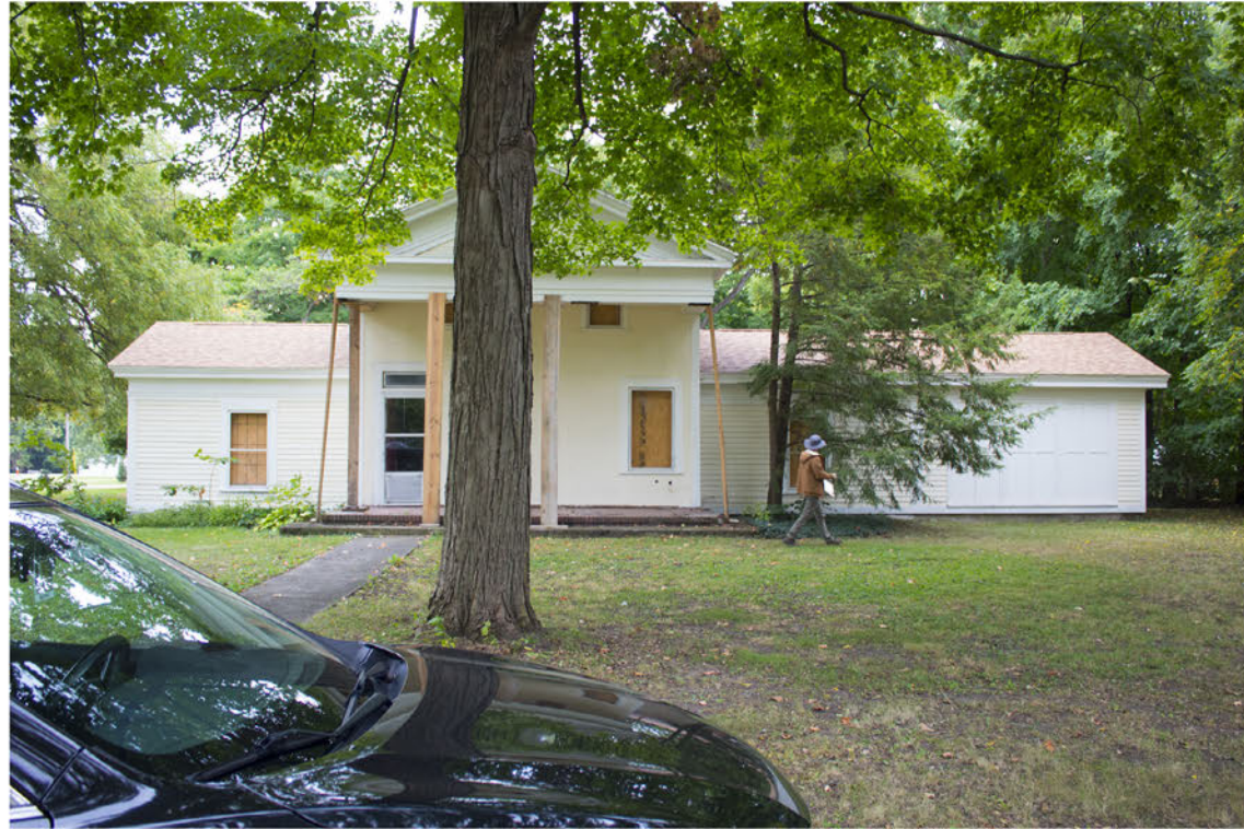
Photo of the current condition, the metal siding was removed and the previous wood one was exposed, in the right wing a new one has to be placed.
