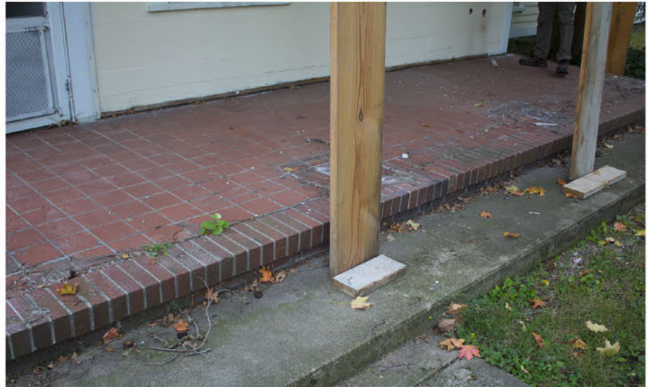
It is described in the National Register of Historic Places Form of the Howe Mansion that in 1958 “the wooden porch floors and steps were replaced with concrete and bricks” , probably both works were undertaken at the same time.
