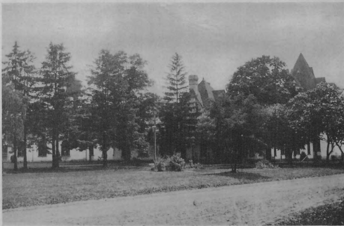
NORTHEAST VIEW OF THE MAIN BUILDING.
