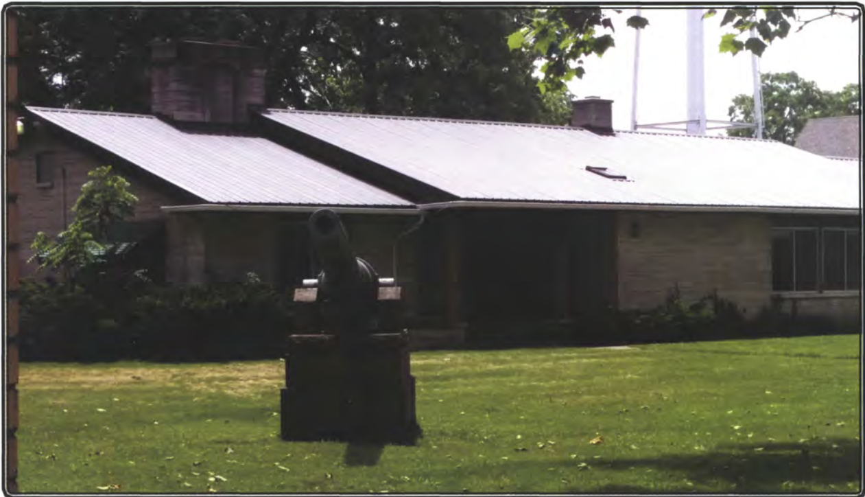
New Metal Roof on the Paul E. Burns President's Quarters
