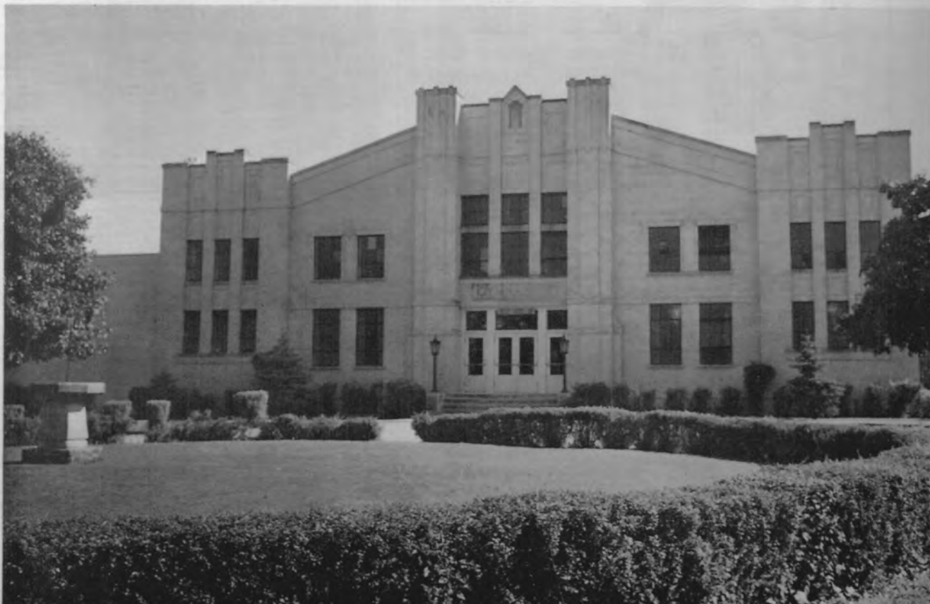
The Gymnasium and Pool
